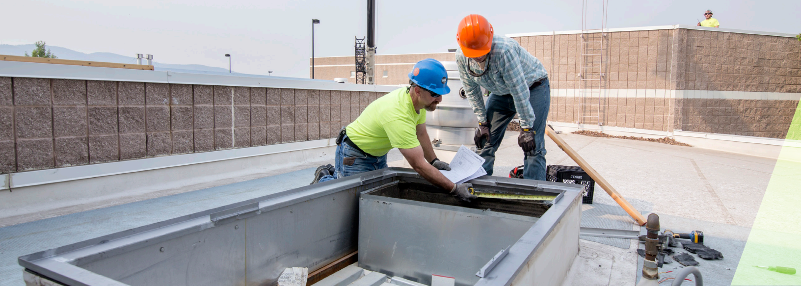
Post Falls, ID — On-site planning ensures proper placement of condensate line.
