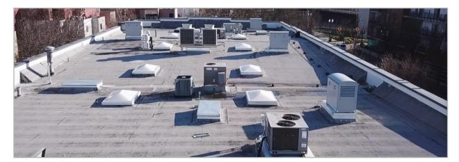
[Figure 1: Very High Efficiency DOAS installed on rooftop in Portland, Oregon]
